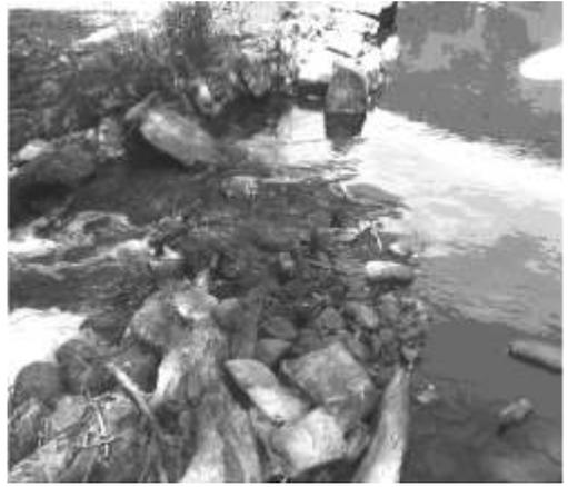
*Dulverton Weir section showing flat facing stones (now buried under the temporary repair)*
